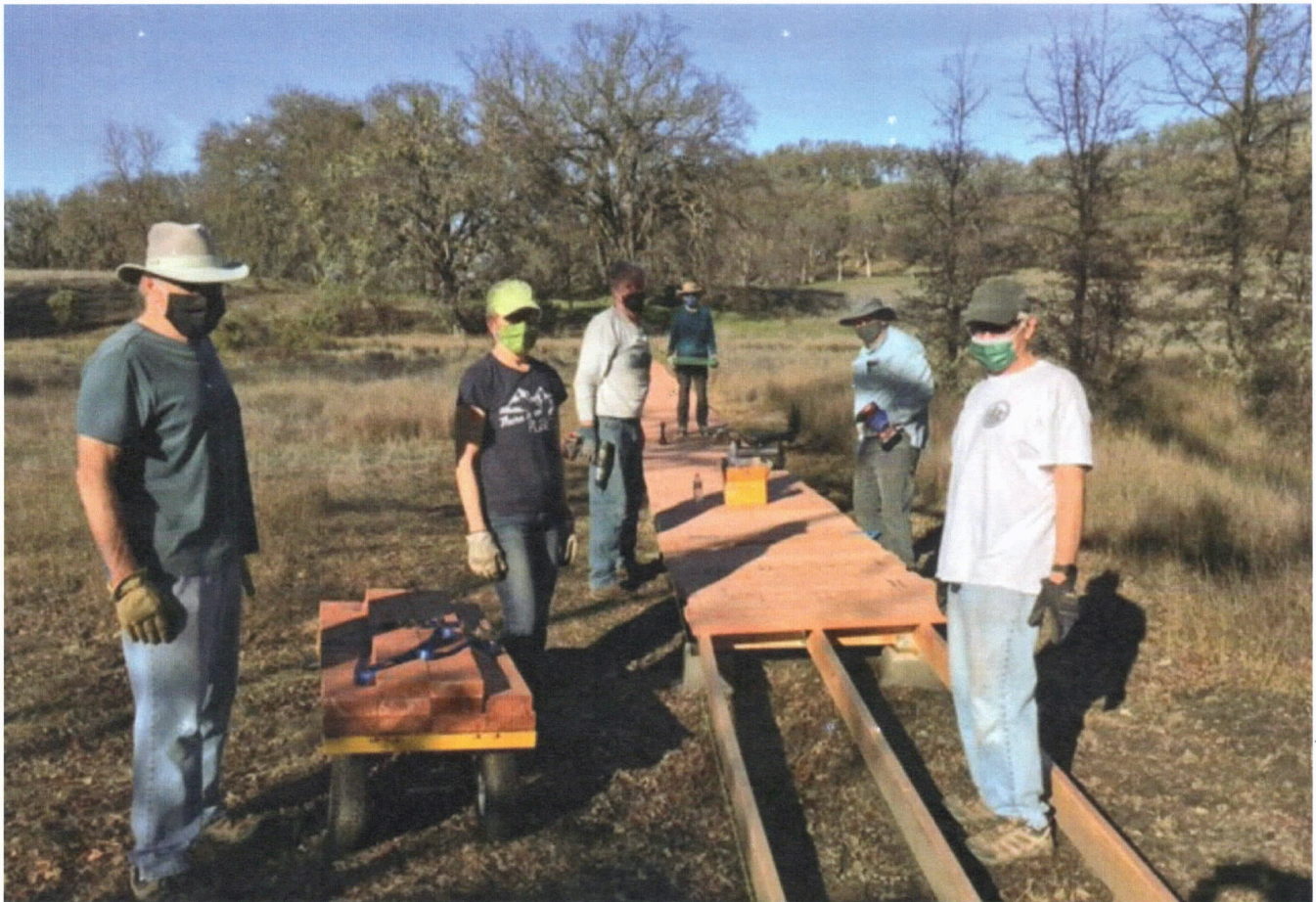
Volunteers at work hammering the final boards on the new boardwalk last winter.
