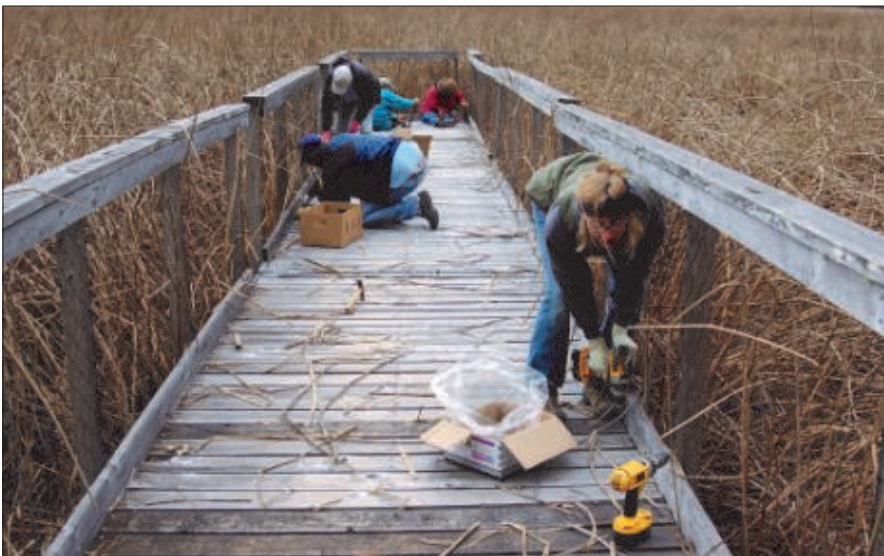
There was a good turn out for the November work party at the Boggs Lake Preserve. Several jobs were accomplished, including pulling all of the old nails out of the pier and replacing with screws. Pictured here is executive director Catherine Koehler drilling in the screws as other volunteers pull nails.
